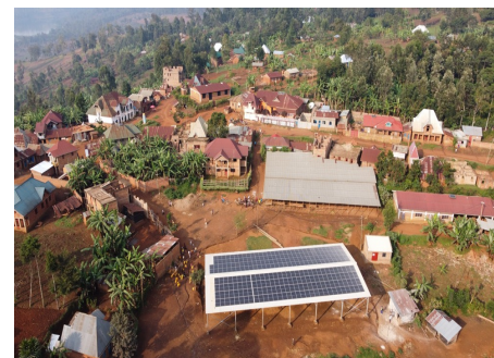
Impianto Off-Grid a Kashara, Congo (2021)
